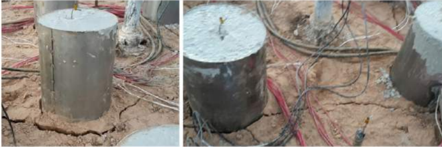
Figure 13. Photographs of cracks in ground surface at a corner pile and at two side piles.
