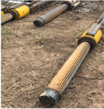
Figure 3. Photo of the EBs and BD before pile construction.
